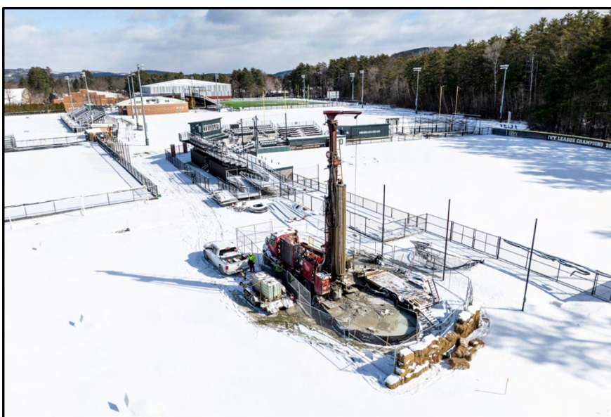
A geo-exchange test well is drilled on Dartmouth's athletic fields. Several CFI grants were awarded to support faculty campus as lab research on the bore fields planned for 2025. Photo credits: Chris Johnson.
